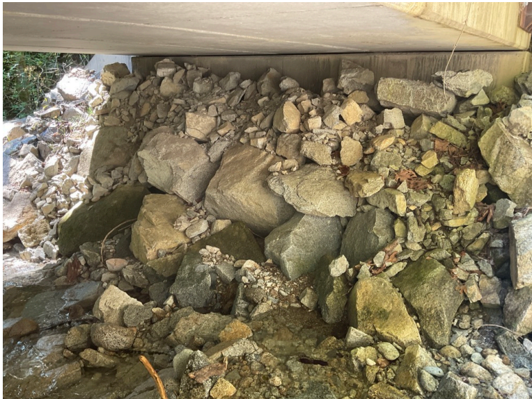
Right Bank Abutment when facing downstream
