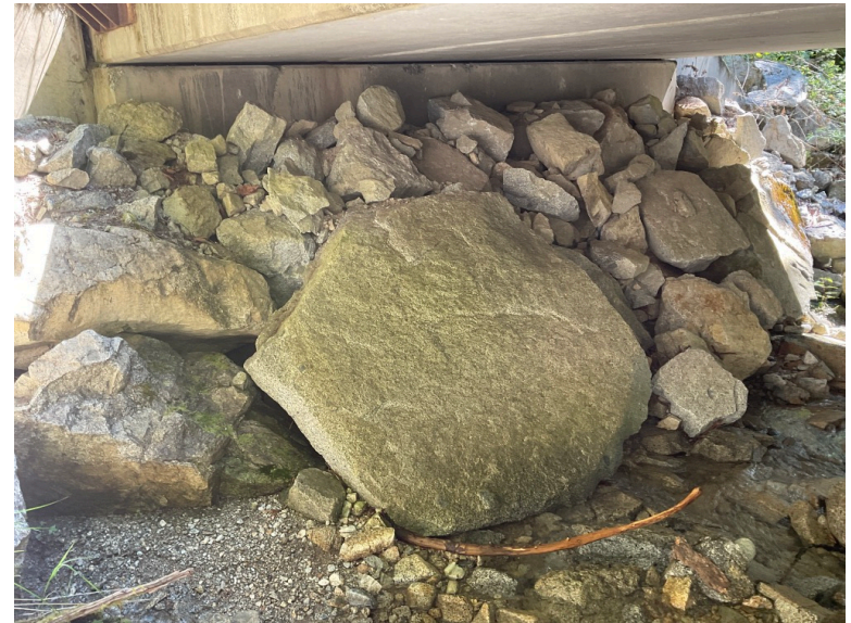
Left Bank Abutment when facing downstream
